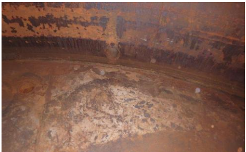
Tank Internal Inspection
