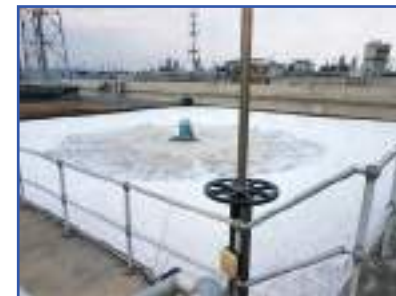
Figure 3a: Aeration tank covered with "foam". This can be caused by the illegal discharge of certain heavy metals, which inhibit the biological treatment process and the breakdown of detergents.
