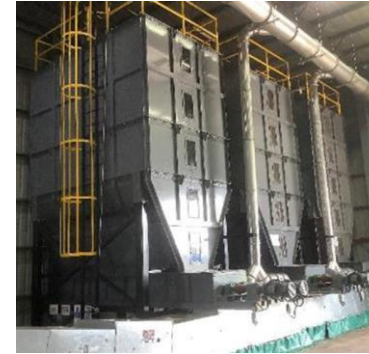
Silo storage bins
