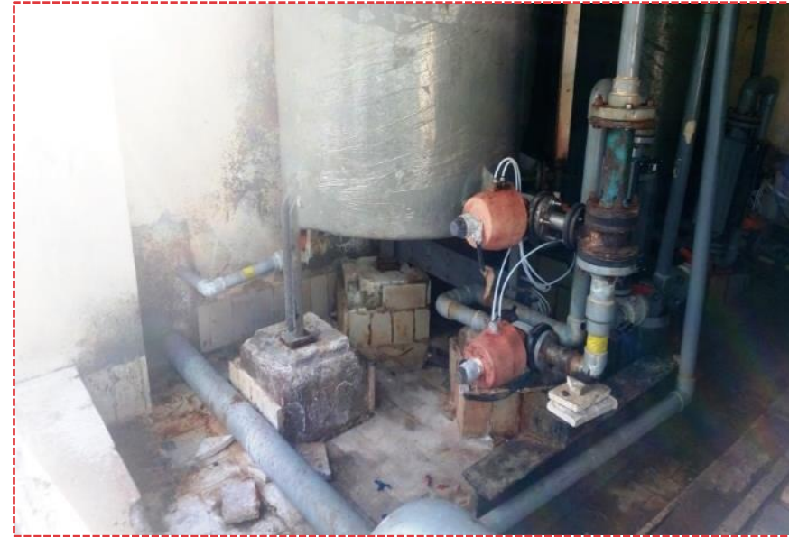
Acid system support integrity
