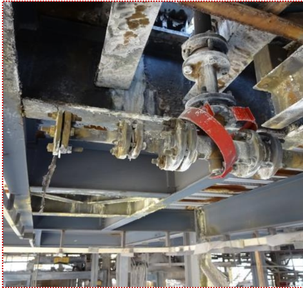
Improper flange guard Uneven bolting
