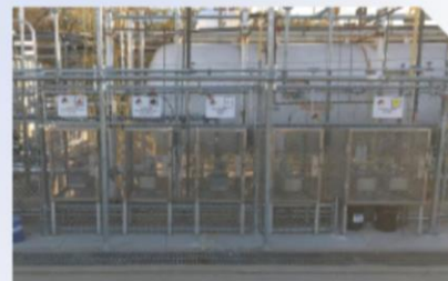
AFTER: New unloading portals with magnetic key fob access (photo courtesy of MGPI)
