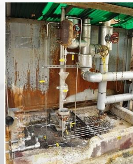
Tesoro Martinez Refinery | Martinez, CA February 12 / March 10, 2014
