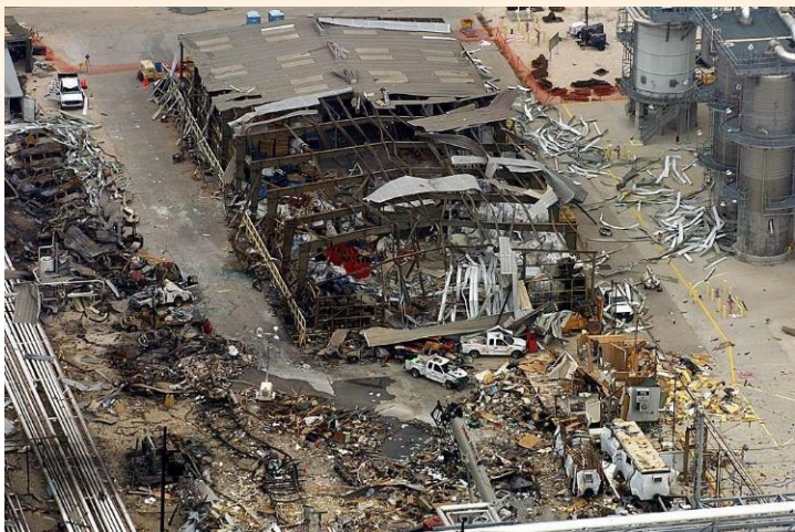
BP America Refinery | Texas City, TX March 23, 2005
