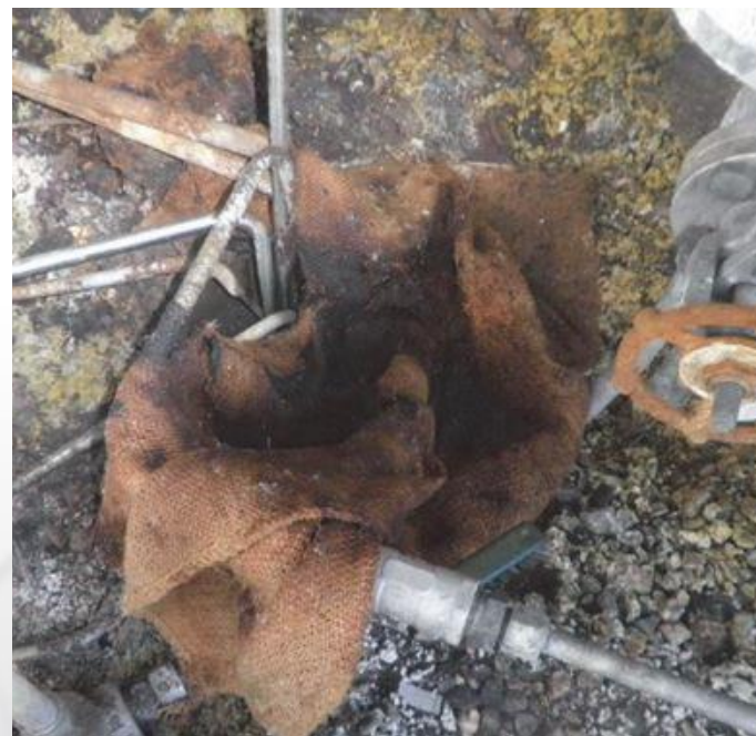
Burlap bag covering the process sewer drain
