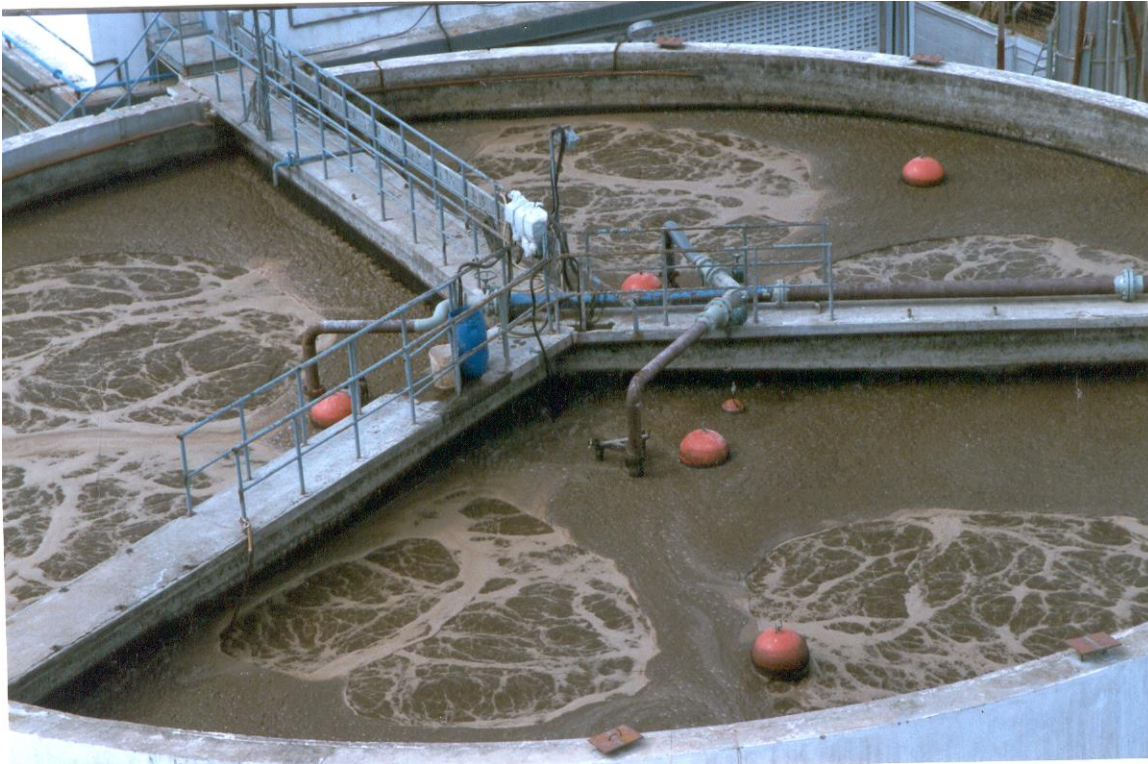
Effluent Aeration Tank
