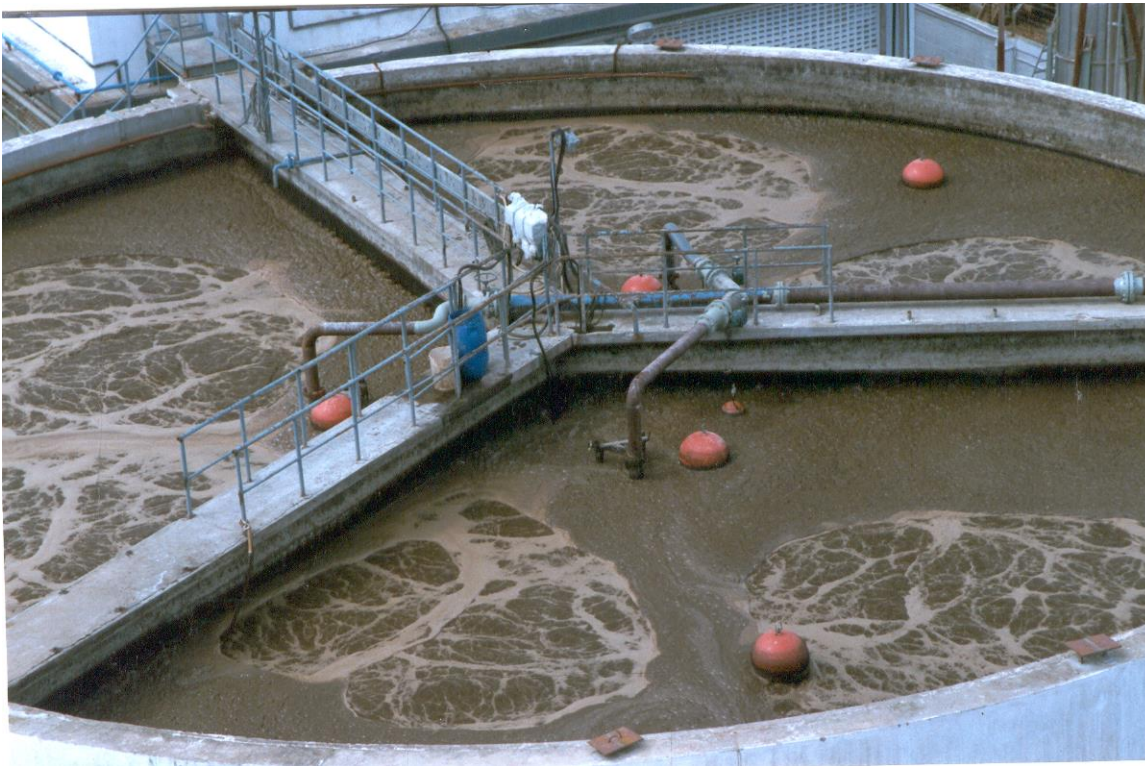
Effluent Aeration Tank
