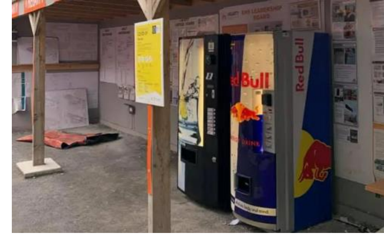
Vending machine onsite
